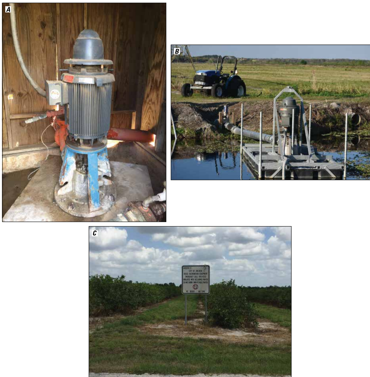
Figure 10. Various agricultural irrigation water sources observed in Florida between 2013 and 2021: A , groundwater well in Alachua County, Florida; B , surface-water intake from canal in Orange County, Florida; and C , reclaimed wastewater use in DeSoto County, Florida. (Photographs by Richard L. Marella, U.S. Geological Survey.)
