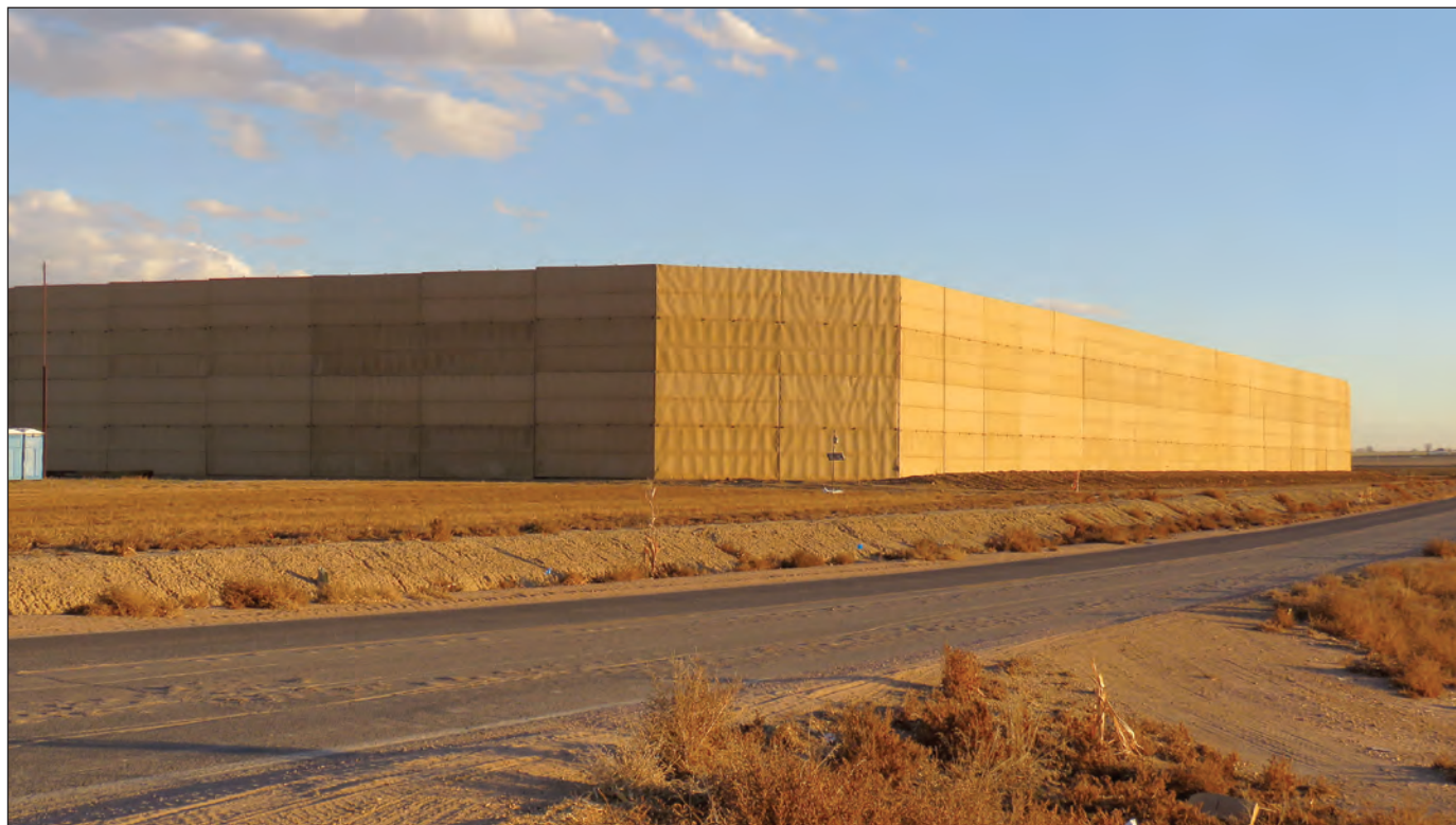
Figure 6. A, Metal sound dampening walls around a natural gas compressor in Colorado. B, Taller padded sound barrier around a well pad in Colorado. [Photographs from Tait Rutherford and Patrick Anderson, U.S. Geological Survey.]
