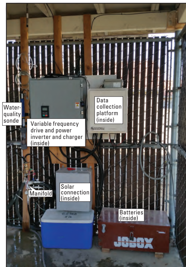
Figure 9. Instrumentation shelter and equipment configuration at multiple well station USGS 364200119420001, 364200119420002, and 364200119420003, Fresno, California.
