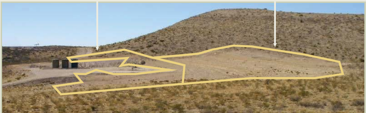
Photograph showing interim-reclaimed areas, differentiating between the area that will be re-disturbed during final reclamation and the area that will not be re-disturbed during final reclamation. Note, there is no stockpiled soil. Photograph by Bureau of Land Management.
