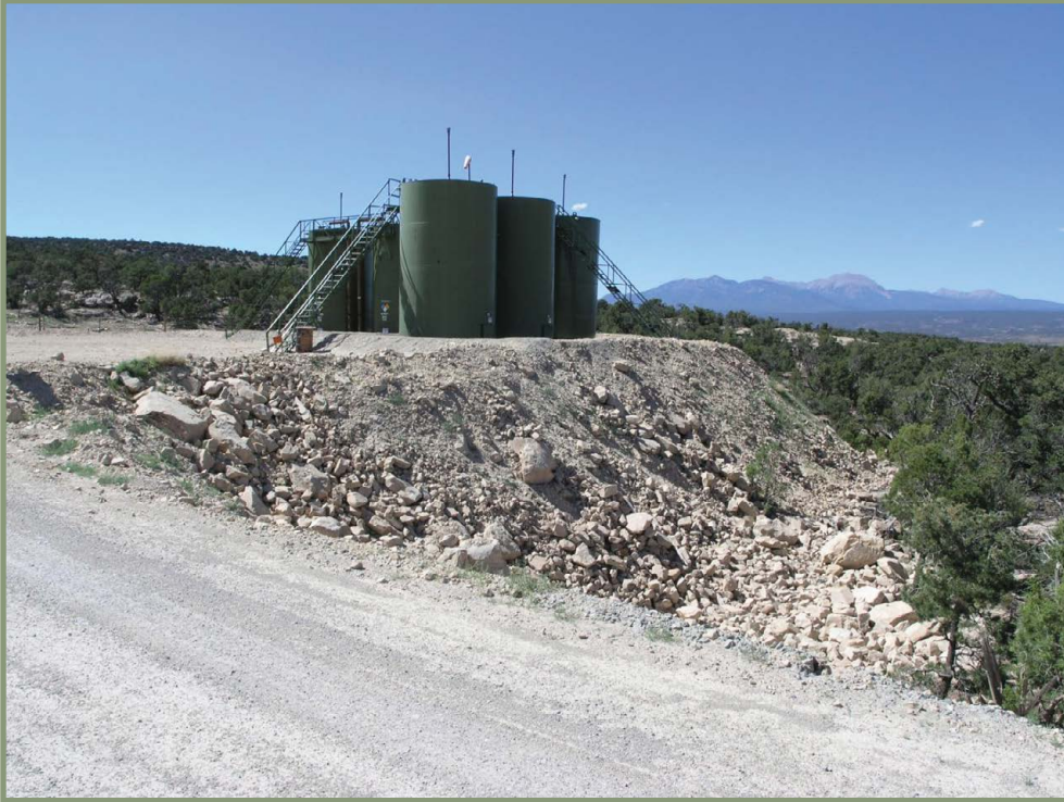
Photograph showing tanks placed on fill. Infrastructure placed on the fill or in the cut prevents recontouring of the site during interim reclamation. Photograph by Bureau of Land Management.
