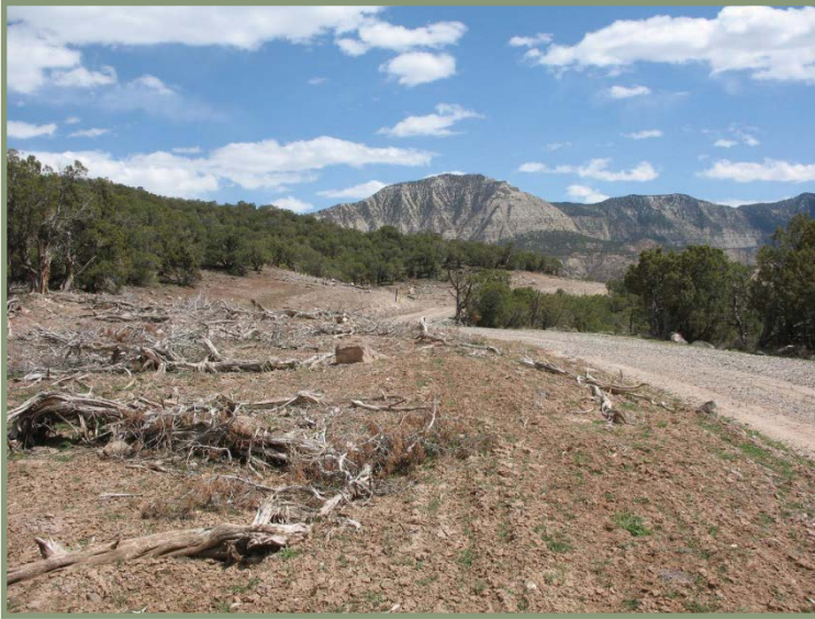
Photograph showing woody plant material used to provide texture and armoring, keep vehicles off the reclamation area, trap soil movement, and create micro-sites for vegetation. Photograph by Bureau of Land Management.
