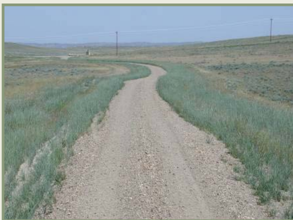
Photograph showing topsoil spread on the sides of roads (in borrow ditches) that has been seeded and maintained to prevent erosion and control weeds. Photograph by Bureau of Land Management.
