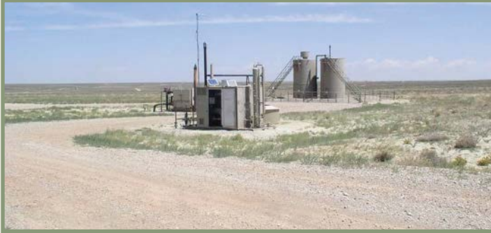
Photograph showing seeding between facilities to maximize the interim-reclaimed area footprint. Interim reclamation occurs as close to facilities as possible, leaving only a small buffer for fire prevention. Photograph by Bureau of Land Management.
