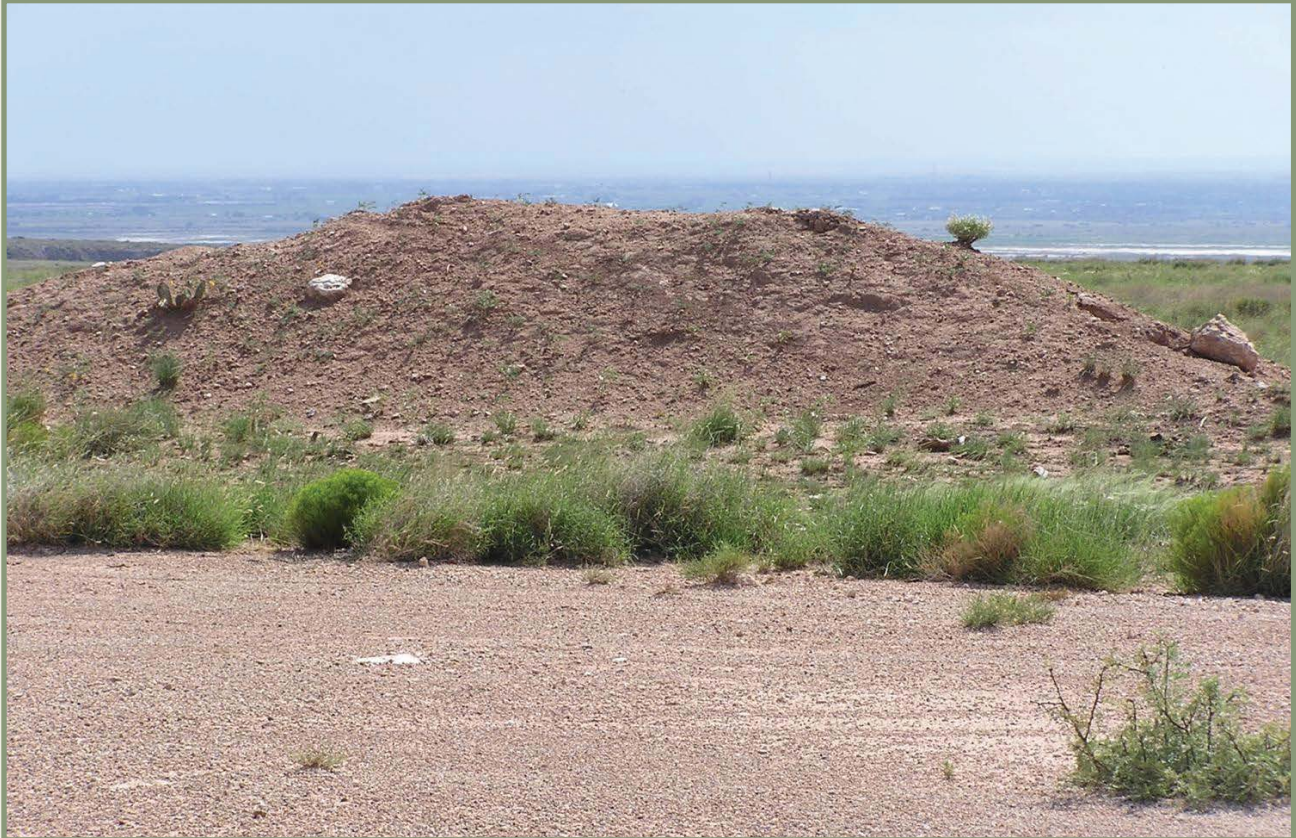
Photograph showing topsoil that has not been handled properly. The pile of topsoil is an insufficient quantity for reclamation and left vulnerable to erosion. Photograph by Bureau of Land Management.
