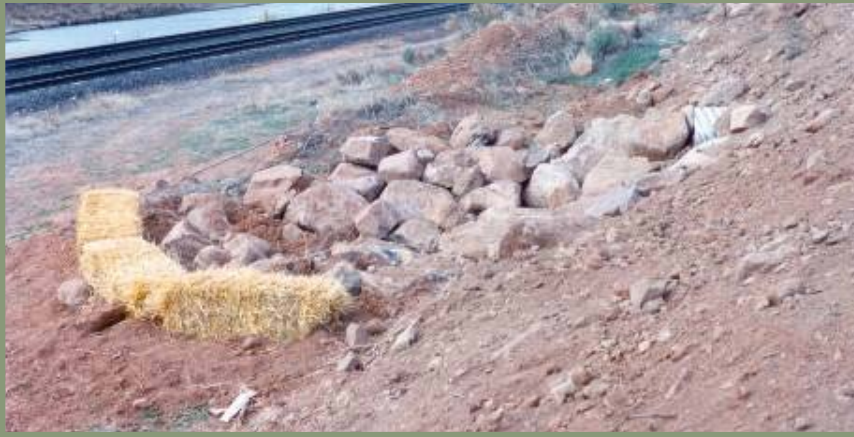
Photograph showing riprap and straw bales used to protect soil at culverts from fast moving water. Note that the rock is sized large enough so that the force of flowing water does not wash it away. Photograph by Bureau of Land Management.
