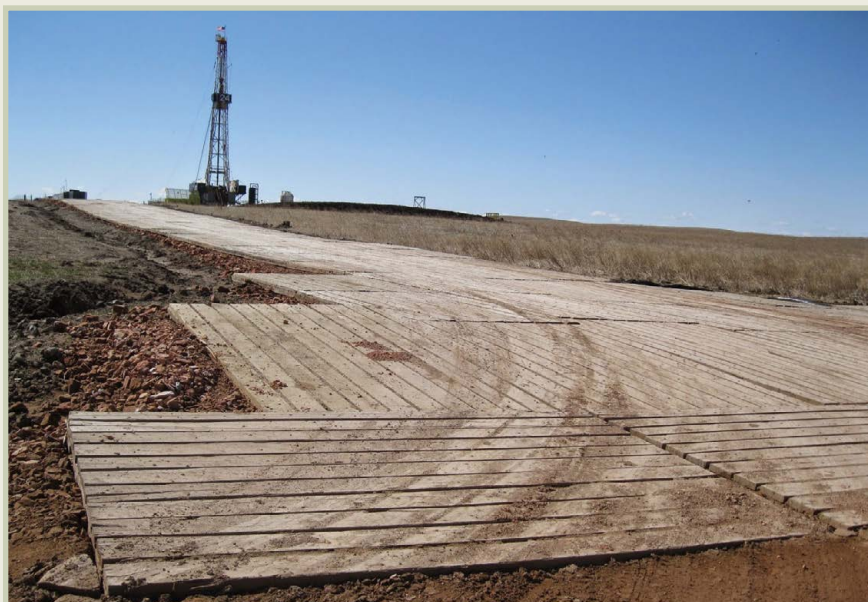
Photograph showing wooden mats laid to access a well, instead of building traditional road and well pad infrastructure, to minimize disturbances to soil and plants. Photograph from Mitchem and others (2009).
