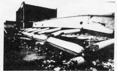
**18** This modern school building collapsed at El Asnam. This school is one of 85 that collapsed during the earthquake. The earthquake occurred after school hours, and so no loss of life was sustained at this school. Photo Credit: Stanford University (H.C. Shah).
