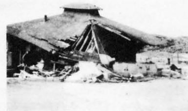
**10** The decorative stone entryway at the West Yellowstone Elementary School fell into a heap of rubble during the 1959 Hegben Lake earthquake. The back wall of the school garage had severe diagonal cracks and later was torn down. The west parapet leaned on a tree. Photo Credit: U.S. Geological Survey (R.W. Bayley).
