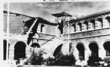
8 The photo shows the west wing of Helena High School that collapsed in the October 31 earthquake. The collapsed part of the school had reinforced concrete frame, floors, and roof, and the tile floors were faced with brick. The greatest amount of damage to a single structure was incurred by this building although it had just been completed only two months prior to the earthquake at a cost of approximately \$500,000. Photo Credit: NOAA/NGDC.
