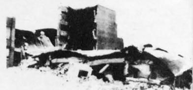
9 The Cummings Valley School completely collapsed. The school building was reportedly constructed in 1910 of concrete walls and a wood roof. The building was a total loss. Photo Credit: NOAA/NGDC.
