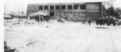
**20** Four hundred children were killed at this elementary school in Dzhrashen southeast of Spitak, Armenian SSR. The precast concrete floors in the building collapsed due to poor ties with the walls. Photo Credit: U.S. Geological Survey (C.J. Langer).
