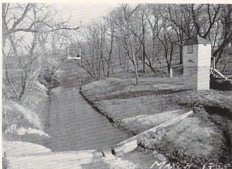
A. ARTIFICIAL CONTROL, GAGE HOUSE, AND CABLEWAY ON RAPID CREEK NEAR IOWA CITY, IOWA
