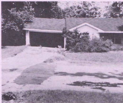
Figure 7. — Photograph of house damaged by a fault in northwest Houston. Fault has deformed garage and has required patch in road.
