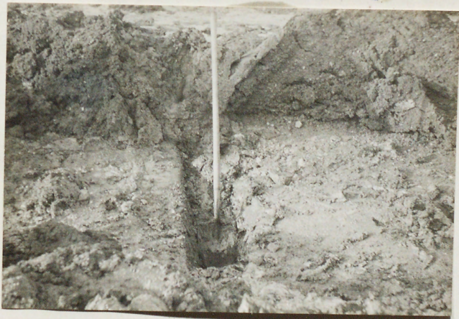
B. FISSURE (INDICATED BY SHOVEL) FILLED WITH LOOSELY COMPACTED, OIL SATURATED CLAY AND BORDERED BY FROZEN CLAY. BLASTING HAS REMOVED THE SURFACE COVER OF PITCH
