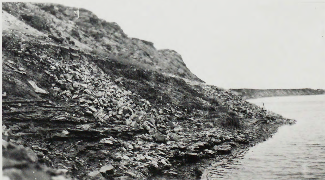
B. Rubble of dense impure limestone from bed about six feet thick overlying thin-bedded sandstone near Meade River coal mine.
