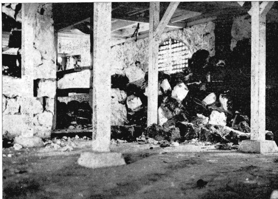
Collapse of partitions in cellar of Puuwaawaa Ranch House resulting from earthquake damage October 5, 1929. Note the wooden posts diagonally braced and footed in concrete, which saved the house when the cellar walls gave way.
