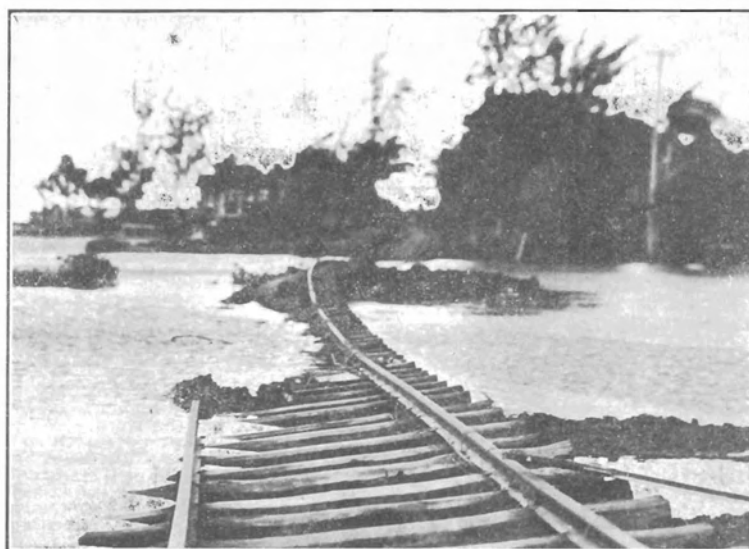
Railroad embankment washed down by tidal wave between Hilo and Kuhio Wharf February 3, 1923. The major wave at Hilo was the third noticed visually, and the waters rose over 20 feet in places damaging wooden houses and wharves. Damage was done also at Kahului in Maui.
