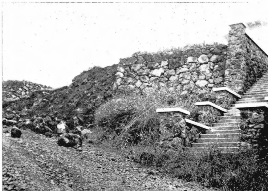
King residence, Honokahau, after the earthquakes of September and October, 1929. The retaining wall of the terrace was shaken down, being built at too steep an angle. Photo Jaggars.
