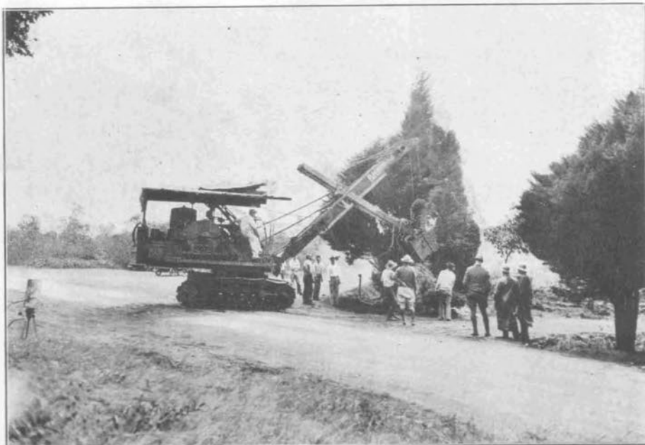
Contractor moving cypress and Japanese cedar trees back from the road front, for purposes of new road construction, Hawaiian Volcano Observatory. Large pits were dug to receive the trees, black fertilizer and loam mixtures were prepared in the pits, and the power shovel with caterpillar treads lifted each trunk with its ball of soil and deposited it at its destination. Photo Jaggar.
