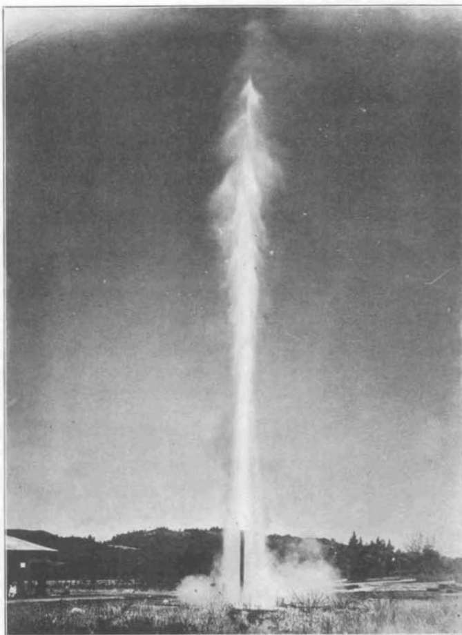
Myrtledale Geyser near Calitoga, Napa County, California. Made artificially by casing a well 180 feet deep, where a stratum containing boiling water is reached. The spouting occurs once every 45 minutes, when the release of steam pressure is satisfied, and it takes another interval to bring the replacement underground water to the boiling point.
