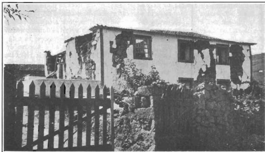
Stucco building damaged by earthquake of August 31, 1926, in Horta, Azores. Photo Agostinho.
