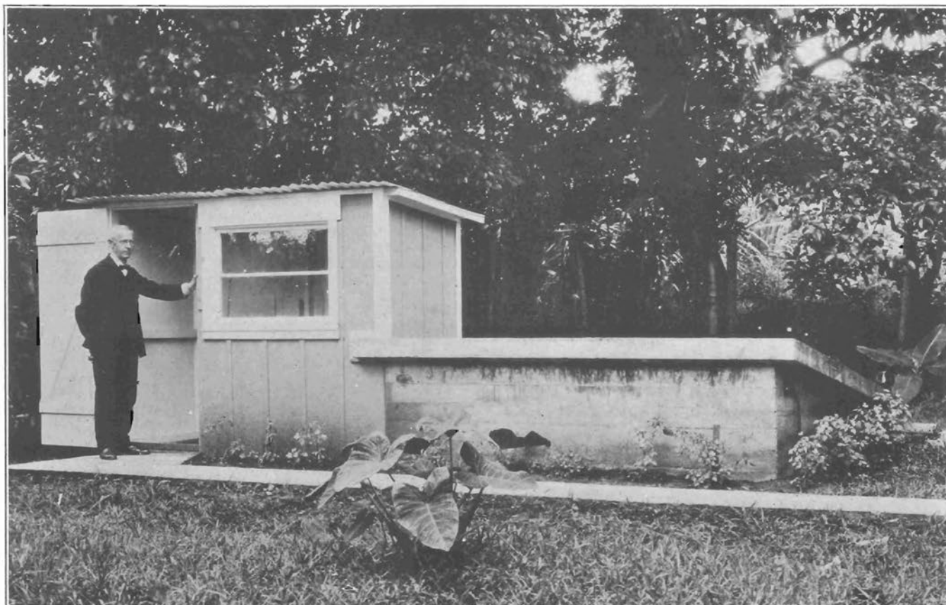
Seismograph cellar of the Hilo station of the Hawaiian Volcano Research Association, built in 1927. Brother J. B. Albert is the observer. The instrument consists of two heavy horizontal pendulums, with clock checked by wireless time signals.
