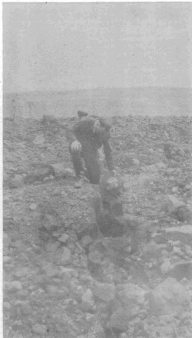
Fig. 3. Rim Crack #46 at point where weekly measurements are made. This crack has continued opening of 4.5 millimeters per week for the past two months.
