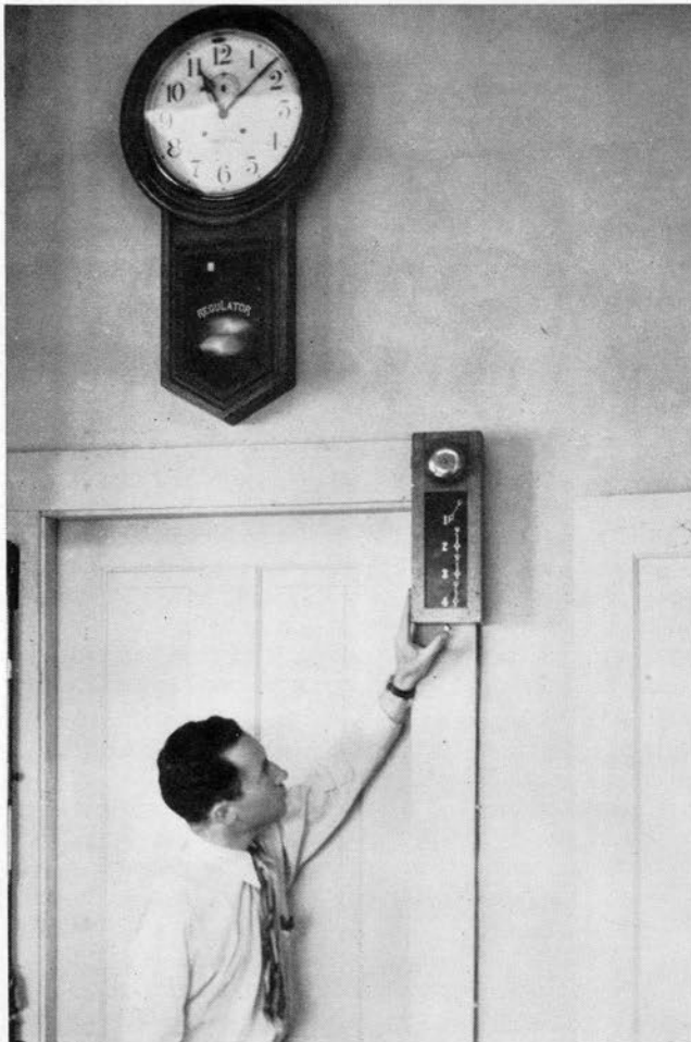
Earthquake Annunciator: Bell and numbers record by arrows earthquake intensities 1, 2, 3 and 4. This notifies the seismologist what the seismographs are doing when he does not feel the quake. Shows also timepiece and mercurial barometer.
