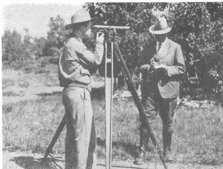
Figure 2. Precise level sighted on a rod marked in decimals of a foot, held upright by a rodman (not shown). Waesche sighting, Jaggar entering notes.
