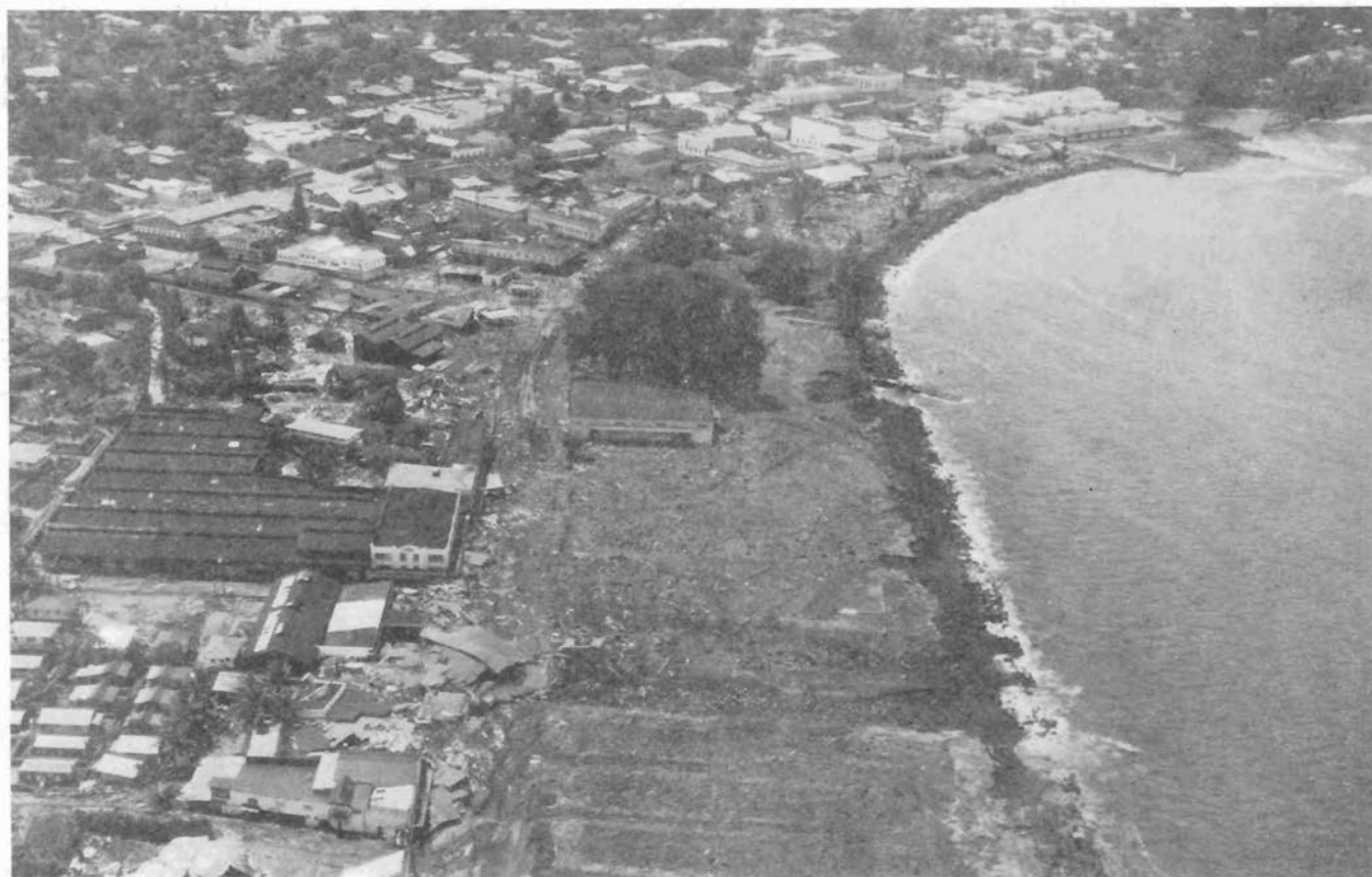
Figure 1.—The waterfront, city of Hilo, April 1, 1946. Two thirds of the railroad bridge spanning the Wailuku River can be seen in the right background. One span was lifted from the piers and carried upstream. The railroad station occupied the barren area on the near bank of the river. The station and the tracks which circled the bay have completely disappeared. All the waterfront buildings between the railroad station and the park (marked by the trees in the center) floated into the street and collapsed. With the exception of the reinforced concrete warehouse, all of the waterfront buildings which occupied the foreground were completely demolished and scattered inland and out to sea.
