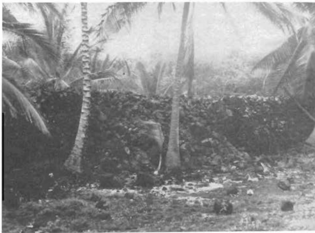
FIGURE 4. Stone wall partly destroyed at the City of Refuge, Honaunau. The wall is approximately 10 feet high. The damaged portion is part of that rebuilt in recent years.
