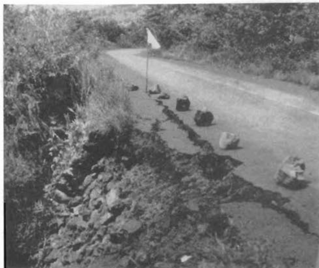
FIGURE 6. Cracking of pavement and slumping of fill at the western edge of the highway near Hookena.
