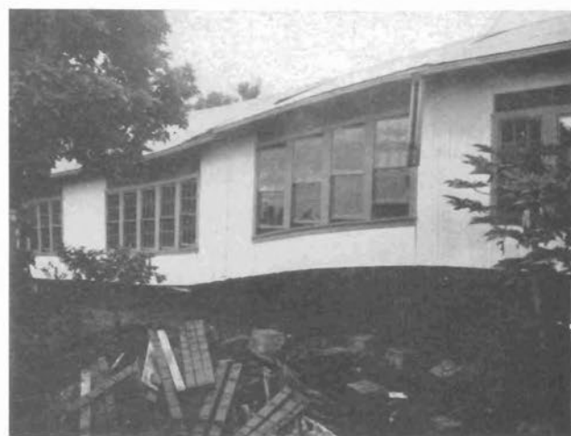
FIGURE 3. Honaunau School. Note the badly deformed window casings, resulting from the earthquake. In the foreground are the fragments of a large water tank.
