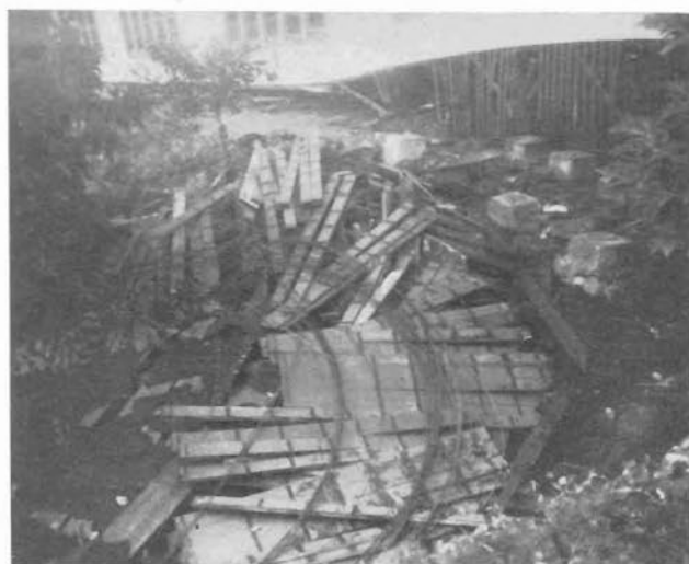
FIGURE 1. Wreckage of 23,500-gallon water tank at Honaunau School. The tank, approximately 20 years old, stood at the southwest corner of the main school building. The concrete footings seen in the background each bore a load of more than 6 tons. The tank appears to have collapsed because of failure of the supporting structure, probably due to inadequate bracing. Photo by G. A. Macdonald.
