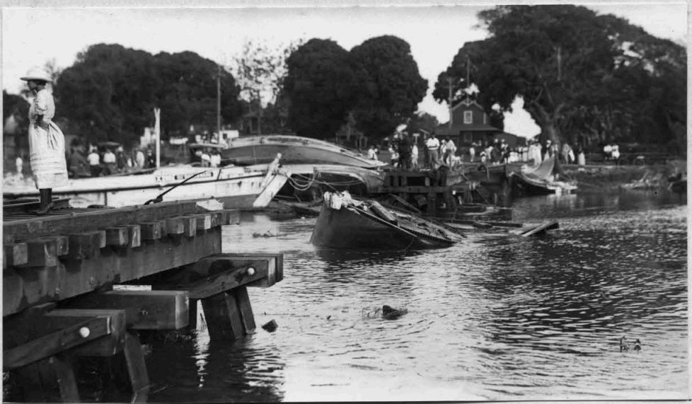
Effects of tidal wave at R.R. bridge across river near Waiakea station
