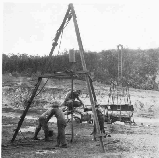
2. Men rotating clay auger. Calyx drill in background.
