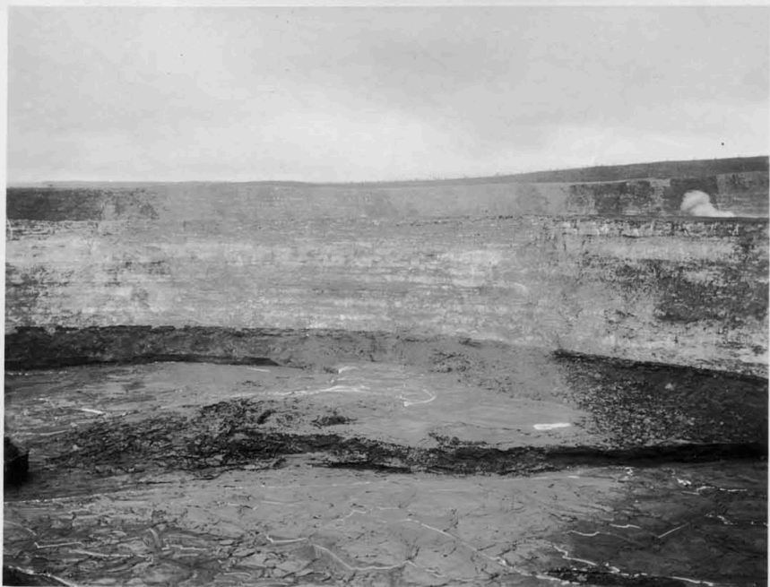
2. Looking northwest from S.E. rim of pit.
