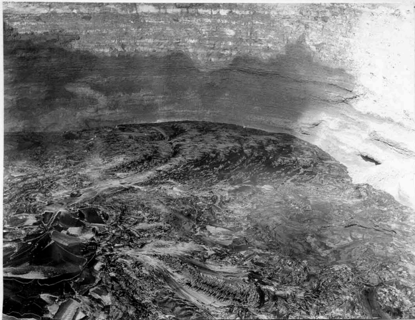
3. Southeast side of pit from S.S.W. station.
