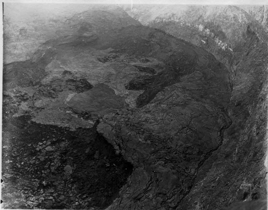
3. South collapse from SW station.
