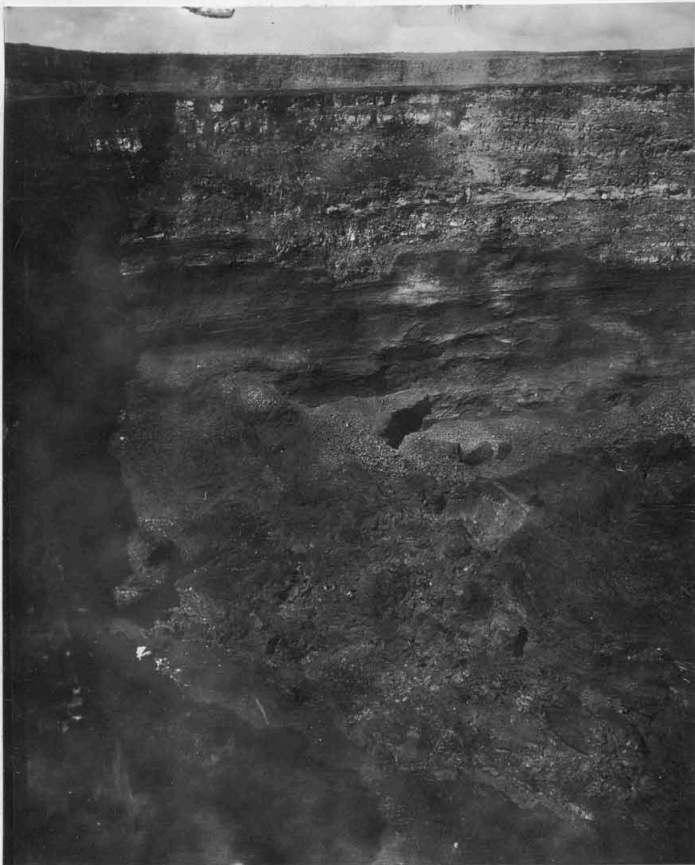
1. Northwest side of pit from S.W.
