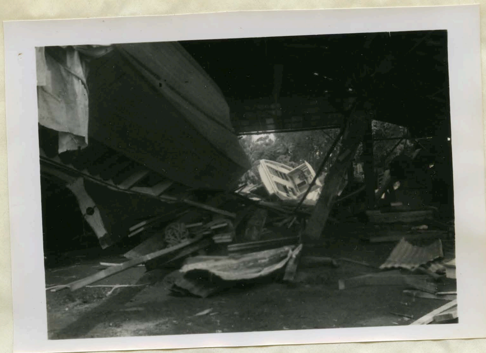
521106-3 Interior of boathouse off Lihikai Street, Hilo, showing derangement after tsunami of November 4, 1952. Ph: Wentworth.
