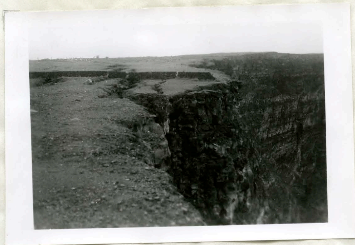
540513-1 0900: Cracks in and near old stone wall at N edge of old tourist overlook area at SE rim of Halemaumau, seen from a point about 250 feet NE of the craterward end of the stone wall. The close end of the rim block in the foreground fell off last night (compare 540512-1 and 540512-2). Ph: G. A. Macdonald.
