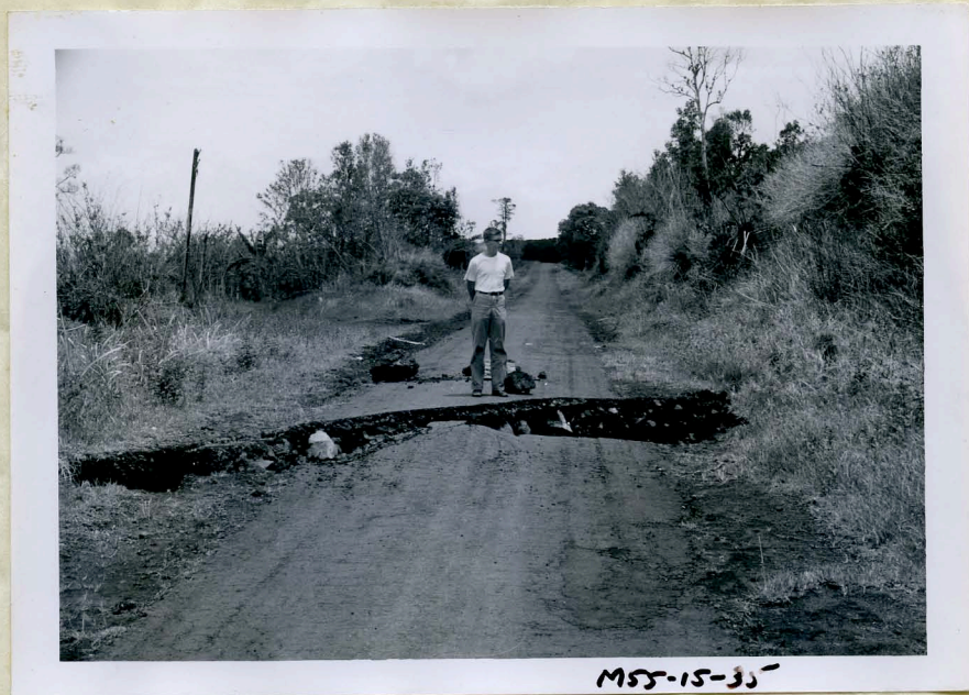
M55-15-35 Fault scarp across old Kalapana Road south of Hayashi's; late June, 1955.
