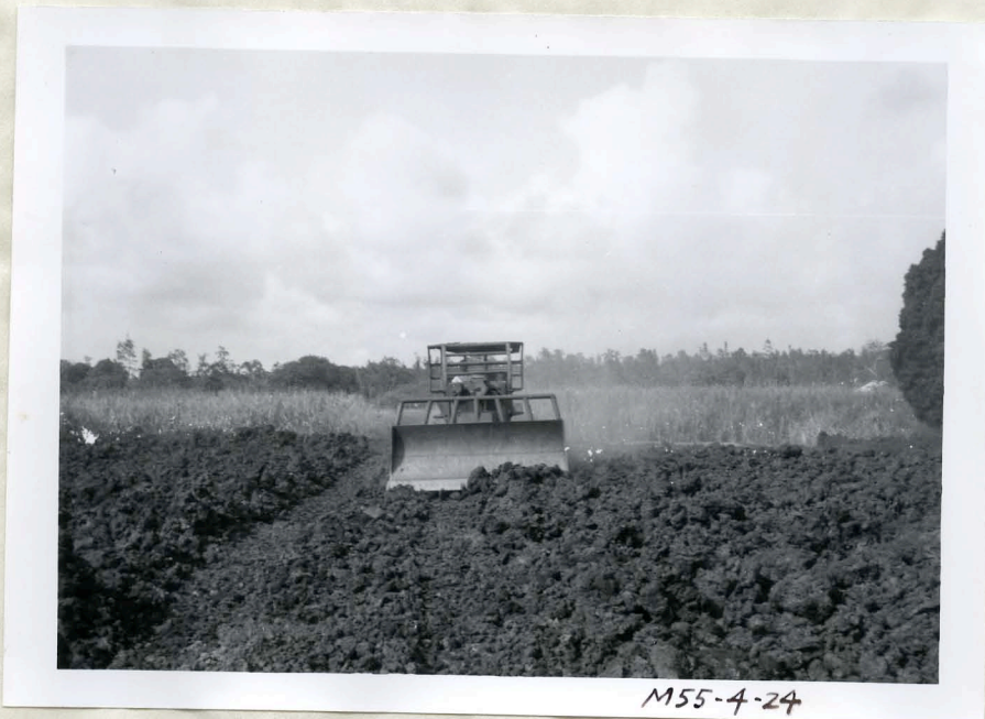
M4-24 Bulldozer cutting new road across Kudo flow; Mar. 20, 1955.
