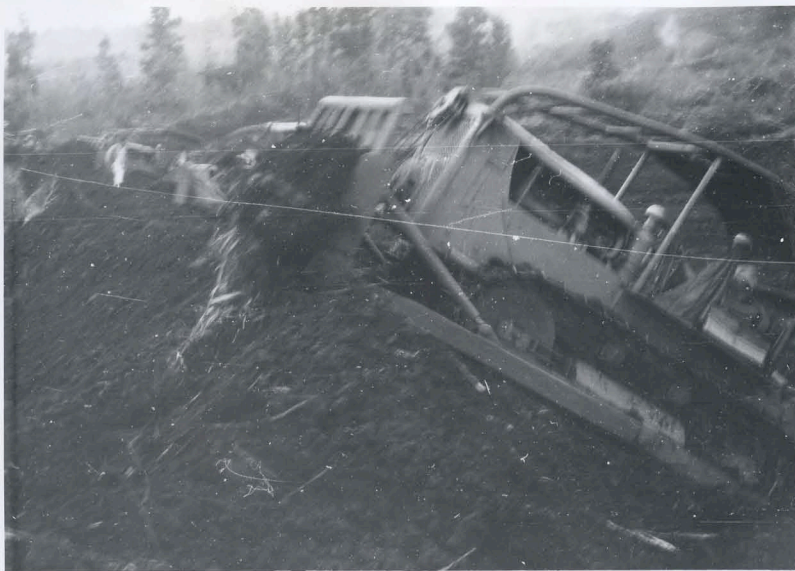
M4-34 Bulldozers building barrier above Iwasaki camp; 13:00, Mar. 21, 1955.
