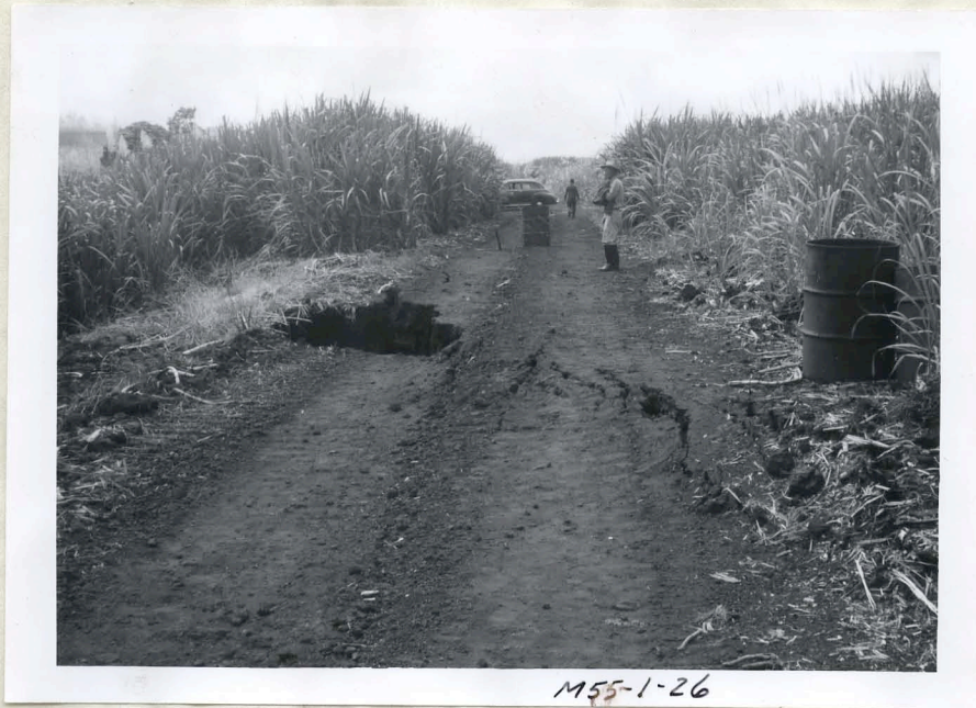
M1-26 Actively developing fault and cracked monocline, on railroad bed road near base of Kaholua o Kahawali hill. Note left side of fissure has caved in since last picture. 12:05, Mar. 2, 1955.
