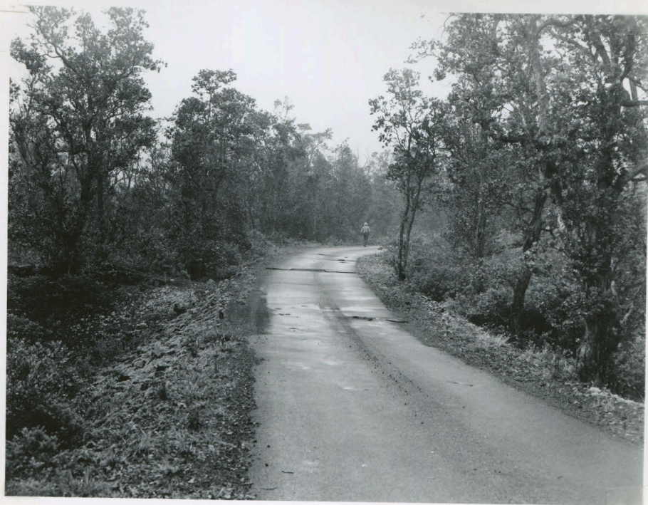
25 Dec 1965 - Cracks Lanakua of Kalihyaa tilt Station (300 yds.)
