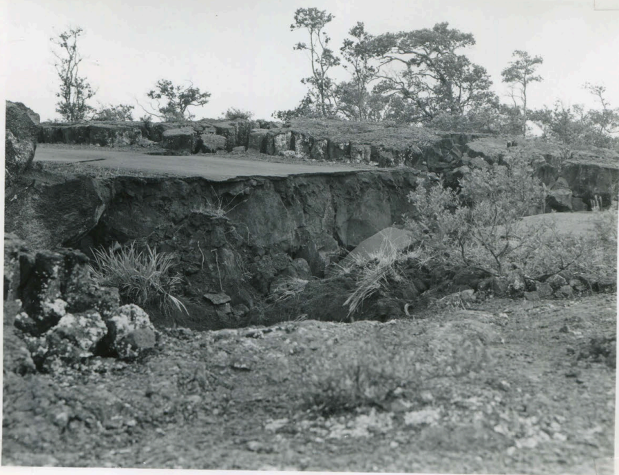
25 Dec 1965. Cracks- Mauna Iki Trail / Helina Pali Road- Ha Povera.
