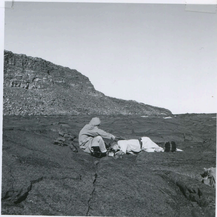
Installing Mauna Loa seismographs Jan. 1964
