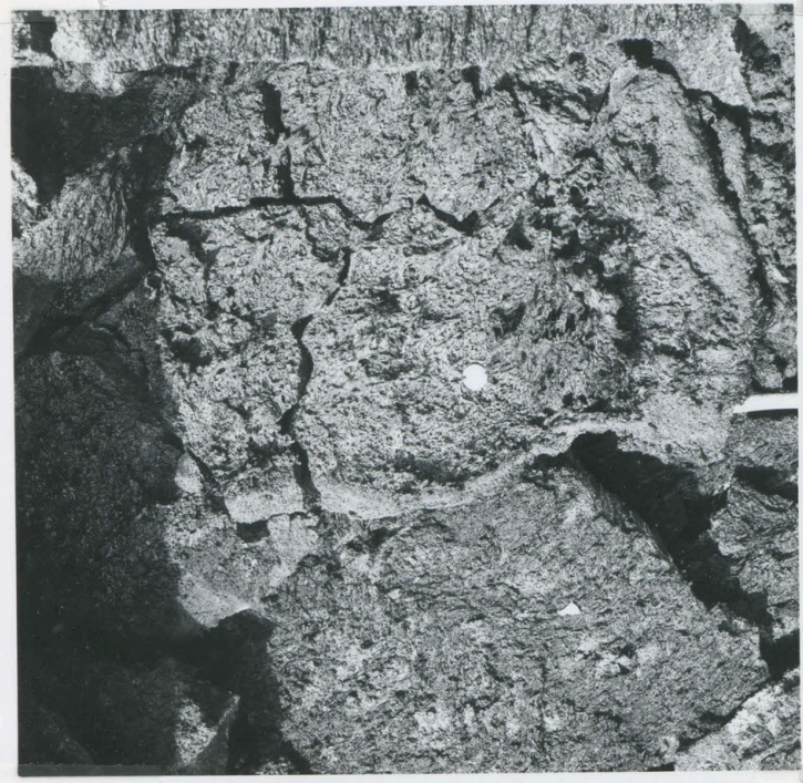
9-63 underside of slab
