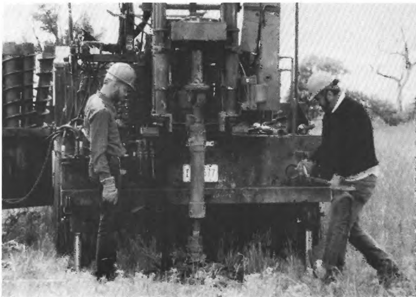
Drilling Observation Well
