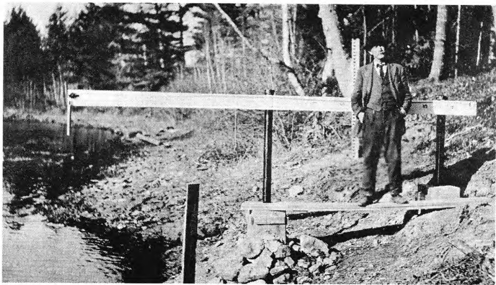
Chain Gage on Passadumkeag River at Lowell 1915
