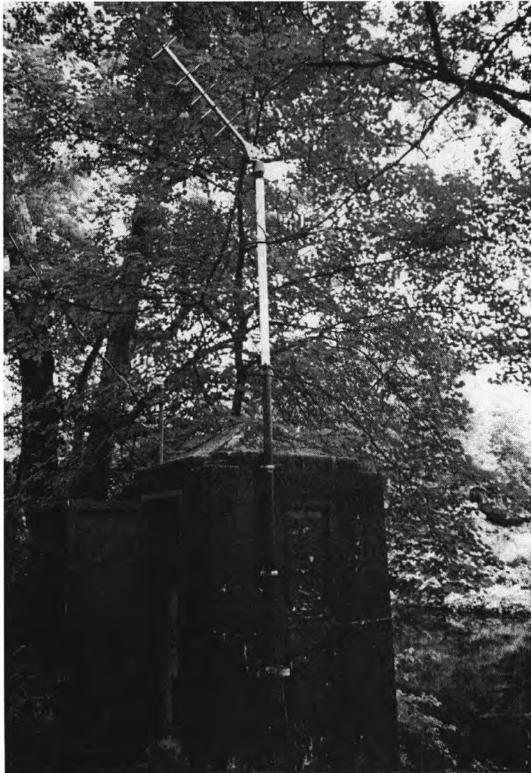
Concrete streamflow gaging station and satellite transmitter antenna, Charles River at Dover, Mass.
