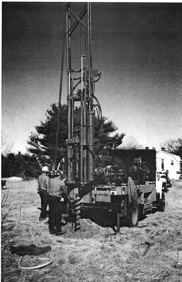
USGS drill rig installing new ground-water-level observation well in Princeton, Mass.
