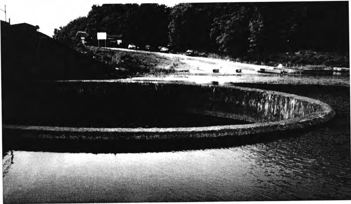
Horseshoe weir showing no flow, Sept. 14, 1995, East Branch Swift River near Hardwick, Mass.
