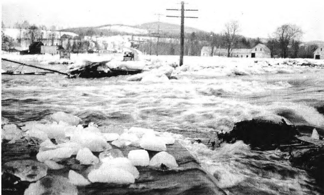
Flood of March 1936 Austin Stream at Bingham, Maine
