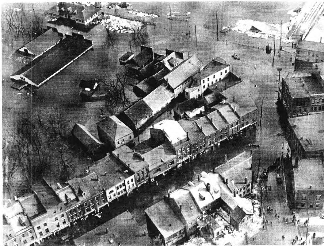
Flood of March 1936 Gardiner, Maine
