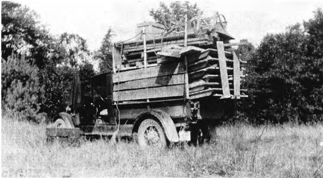
Gage house construction Salmon Falls River near South Lebanon, Maine 1928
