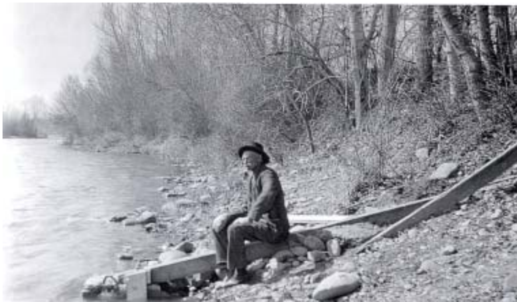
Sloping gage at Salmon River at Salmon, Idaho (April 1924)
