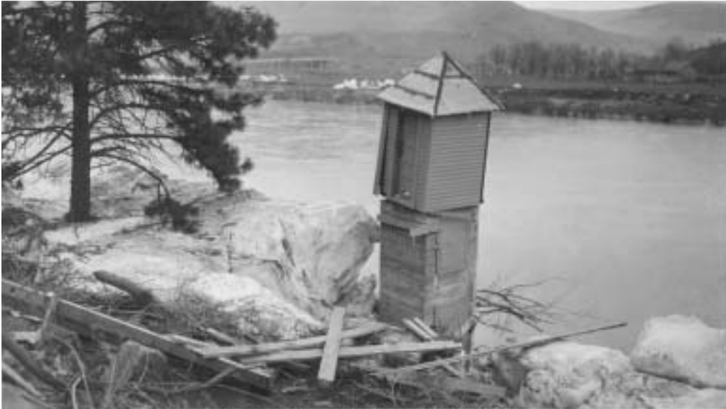
Gage damage following high water at Clearwater River at Spalding, Idaho (Feb. 1928)
