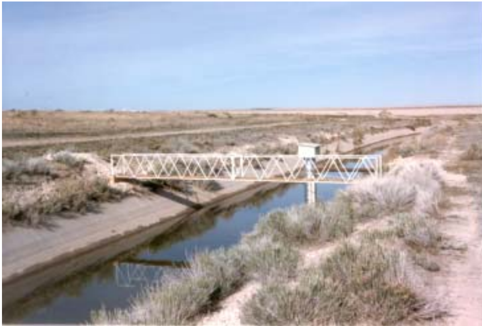
Bell Rapids Canal near Hagerman, Idaho (1985)
