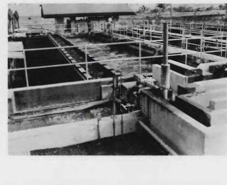
FIGURE 6. PHOTOGRAPH OF SITE 21, KEAHOU SEWAGE-TREATMENT PLANT
