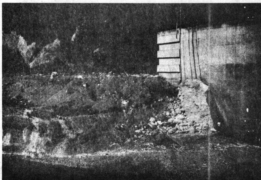
FIGURE 22.--View upstream at Sweasey damsite showing left abutment of dam and remnants of sediment deposited in old reservoir. Man standing on a log at the base of the abutment gives scale. The disturbed concrete and the surface extending horizontally across the left side of the photograph evidence the removed dam and the complete filling of the reservoir with sediment. The Mad River flows from left to right in the left foreground. Photograph by J. O. Armstrong, September 23, 1972. Compare with figure 20.
