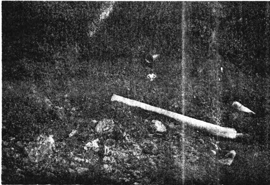
FIGURE 21.--Failure of causeway resulting from channel aggradation about 0.5 mile (0.8 kilometre) downstream from Sweasey damsite. The pipe buried in the causeway was used to transport water from Sweasey Dam to Eureka prior to sedimentation of the reservoir. Man in center of photograph gives scale. Photograph by J. O. Armstrong, September 23, 1972.
