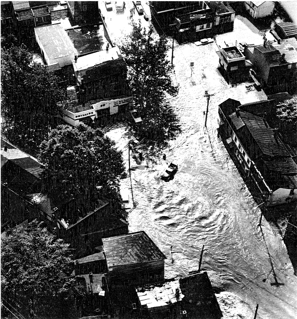
Figure 10.--Intersection of Bridge and Ferry Streets in Trenton inundated by floodwaters from Assunpink Creek which had overflowed onto the main-line Penn Central railroad tracks, July 21, 1975. View is looking east. Trenton Times photograph by Warren Kruse.
