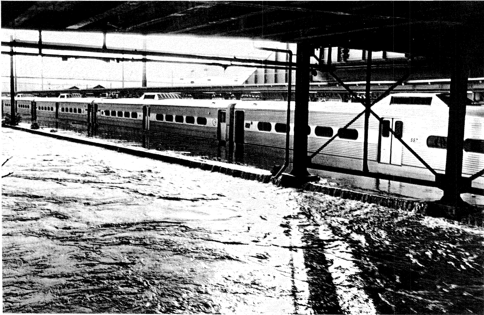
Figure 8.--Flooding along Assunpink Creek under the upper passenger concourse of the Penn Central Clinton Avenue railroad station, July 21, 1975. Trenton Times photograph by Martin D'Arcy.
