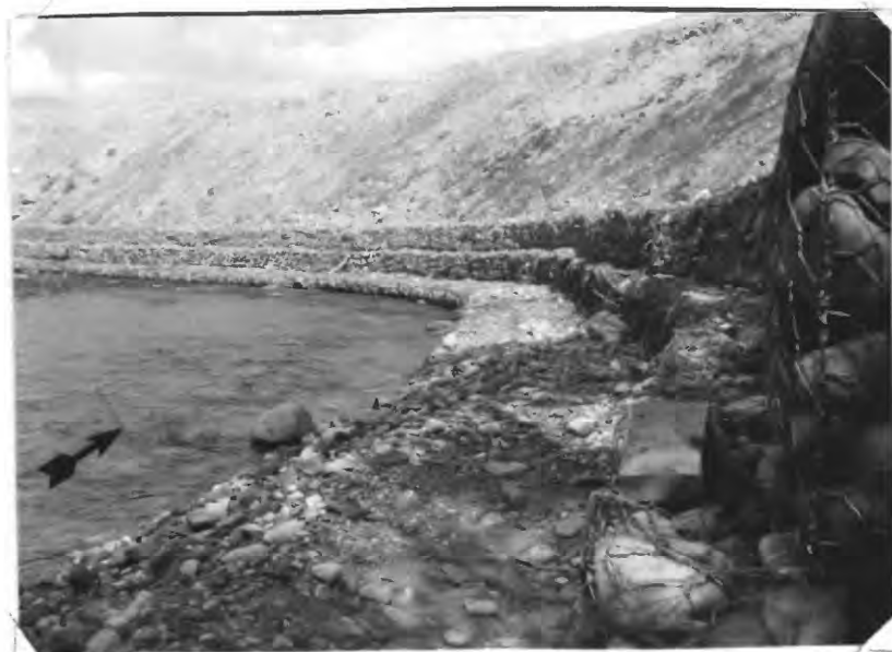
b. View downstream along left bank showing tiers of demonstration gabions. Arrow shows direction of flow.
