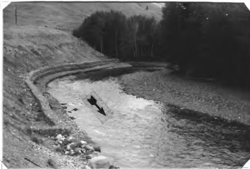
c. View upstream showing lateral extent of gabions along left bank. Arrow shows direction of flow.
