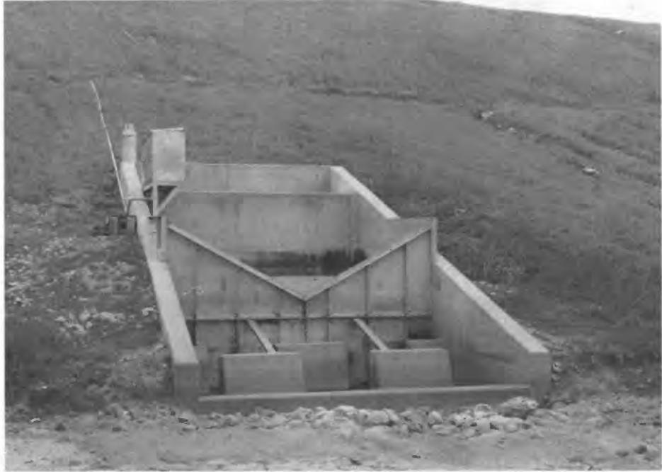
A. Oblique view of control structure
