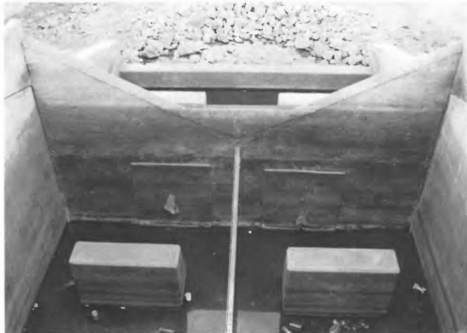
B. Top view of control structure
