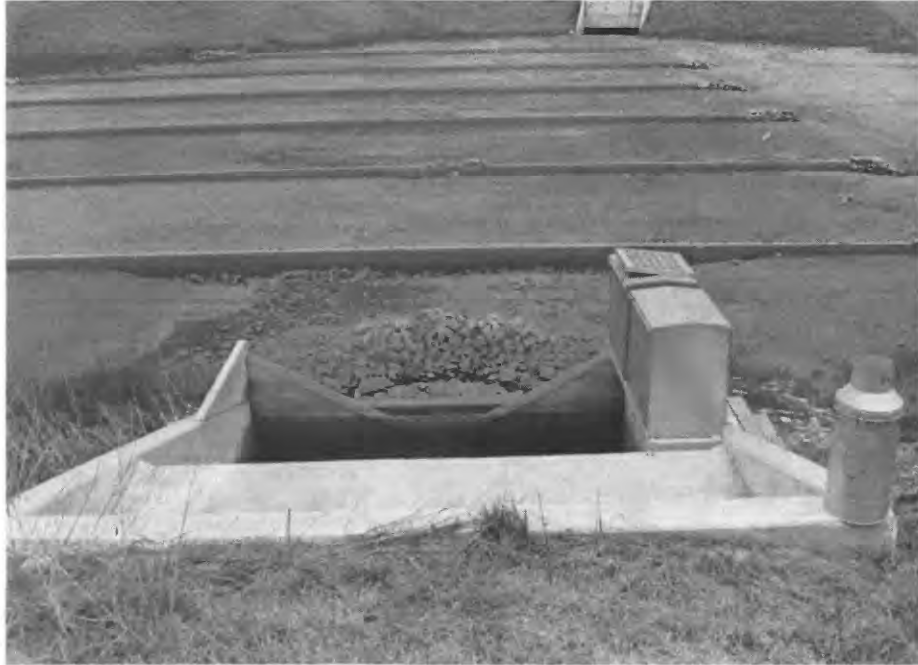
A. Pond 1 at Barton Creek Square Shopping Center
