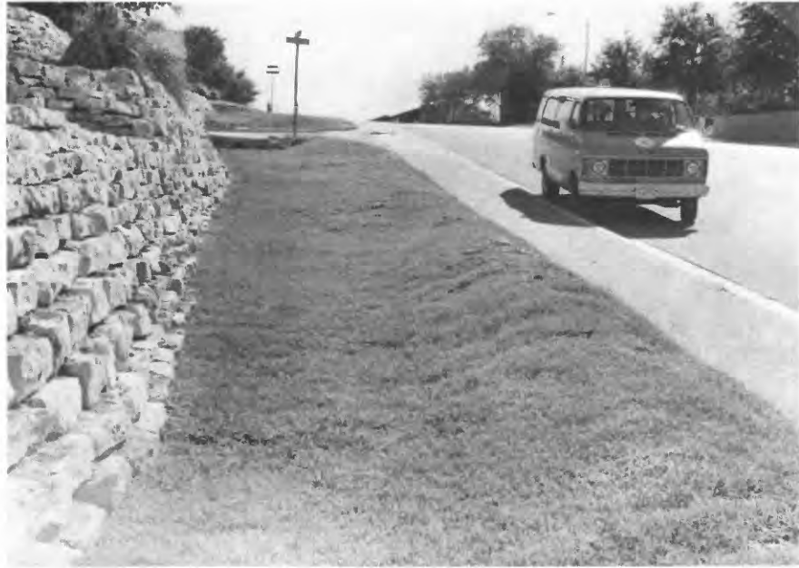
A. Grass swale on west drainage channel
