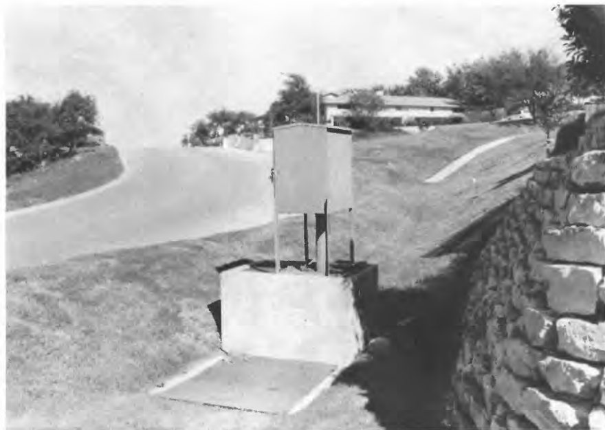
B. Detention pond and outflow gaging station on the drop outlet
