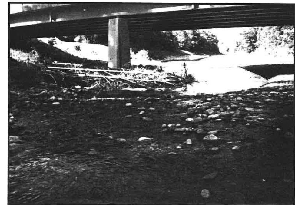
Figure 7. Woody debris accumulation on upstream nose of left (looking downstream) bridge pier at Austin Stream at Bingham, Maine, June 28, 2000.
