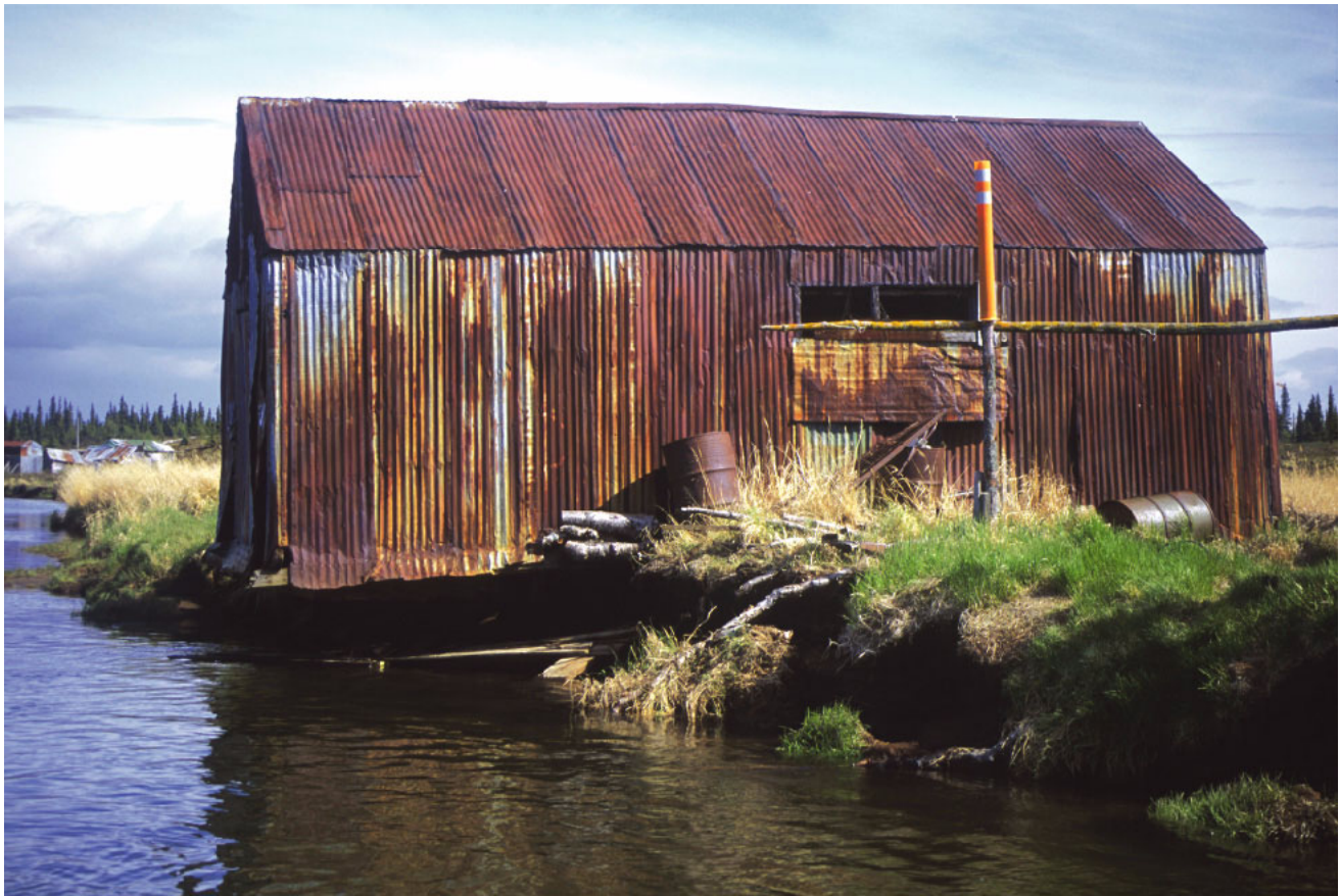
Figure 21. Bank erosion beneath bankside structure, Alagnak River river kilometer 17. Photograph by author, June 5, 2001.
