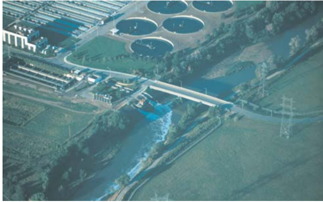
Treated wastewater discharge to the South Platte River downstream from Denver is a source of nutrients.
