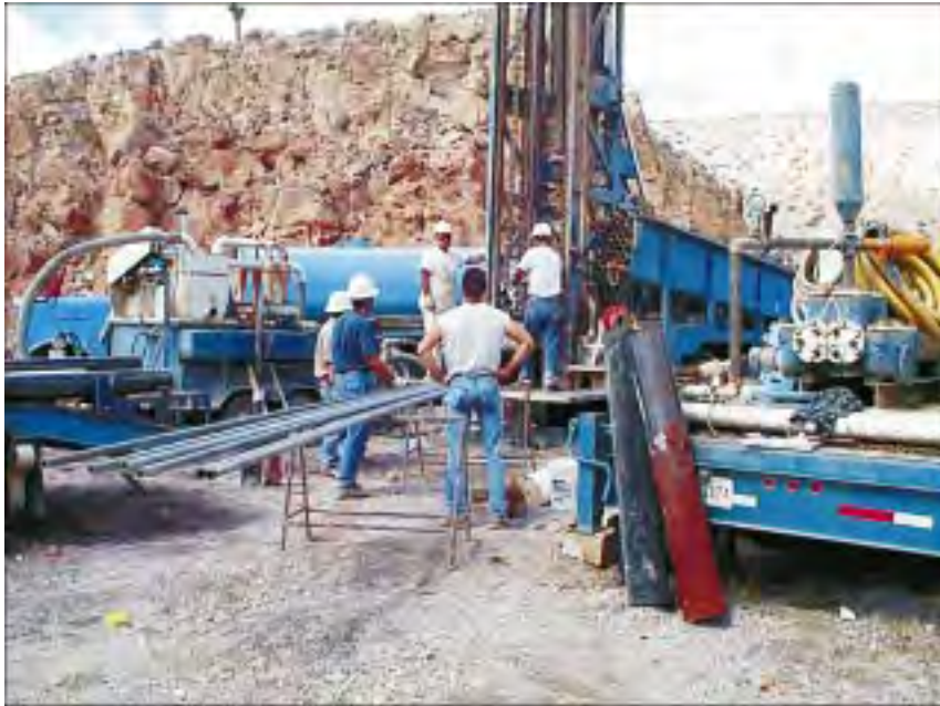
Drilling of well ER-OV-03c near Beatty Wash on the eastern side of Oasis Valley study area (Photograph by Douglas Trudeau, U.S. Geological Survey)
