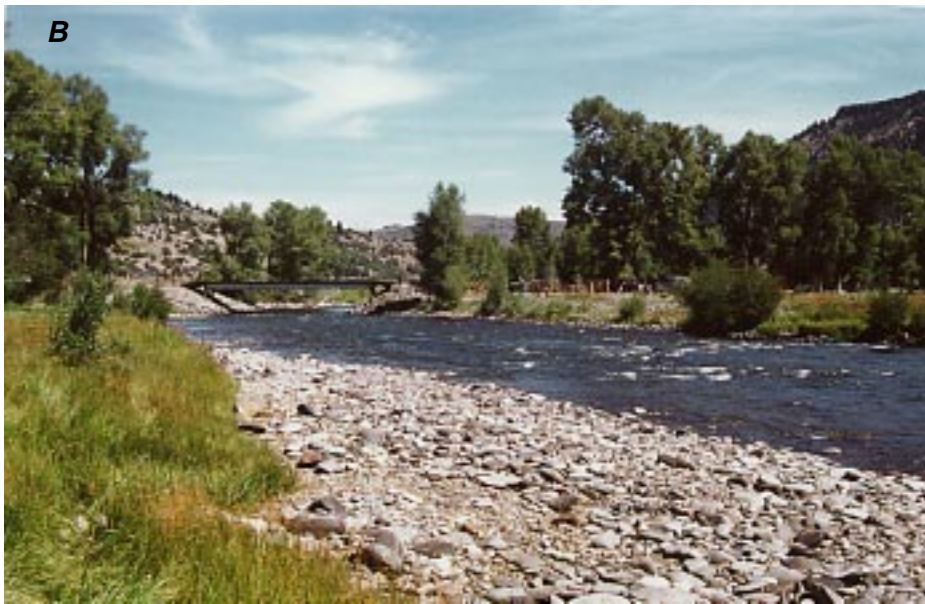
Figure 2. Lake Fork of the Gunnison River at Gateview, Colorado. Views looking downstream to the bridge near gaging station 09124500, (A) in 1992 prior to reconfiguration at a discharge of 270 cubic feet per second, and (B) in 1998 following reconfiguration at a discharge of 230 cubic feet per second. The cobble bar forming the left bank in (B) was constructed of material dredged from the streambed to the right. The large, partly submerged boulders in the right side of the channel in (B) were quarried offsite and added to the streambed during reconfiguration.
