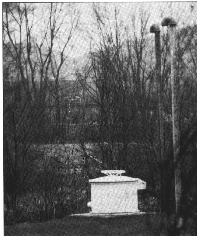
Figure 5. Gravel-packed public-supply well in stratified-drift aquifer in the town of Plymouth, central New Hampshire. (Photograph taken by B.R. Mrazik, U.S. Geological Survey.)
