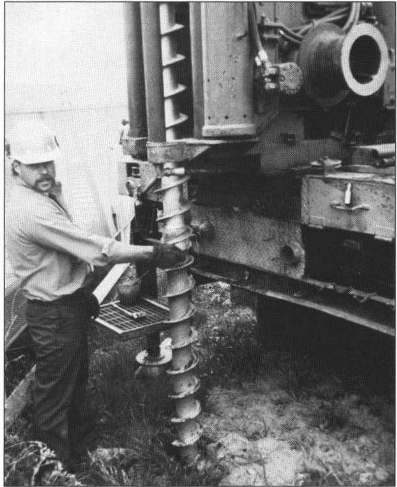
Figure 13. A hollow-stem auger drill rig and operator. This U.S. Geological Survey drill rig was used to drill 674 test holes statewide to collect data on aquifer characteristics and to install observation wells. (Photograph taken by J.R. Olimpio, U.S. Geological Survey.)
