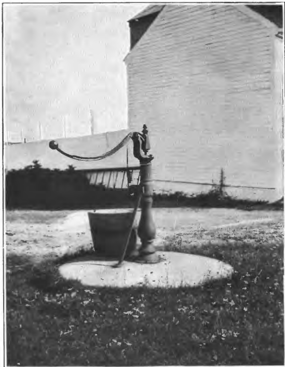
A. WELL AT COUNTY JAIL, WISCASSET. Showing best method of protection from surface drainage.
