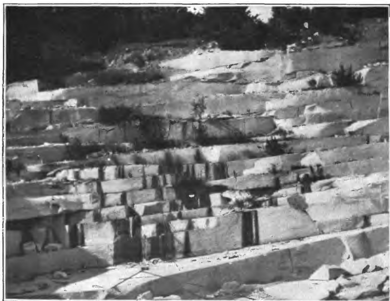
B. VIEW IN CRABTREE & HAVEY'S GRANITE QUARRY, AT NORTH SULLIVAN. Showing occurrence of water in sheet joints.
