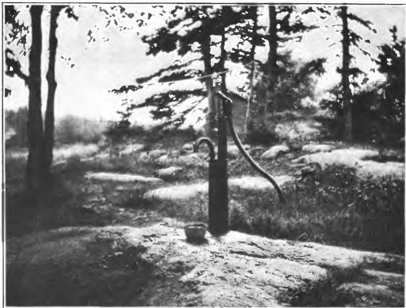
B. COMPLETED WELL BELONGING TO CRABTREE & HAVEY, AT NORTH SULLIVAN.
