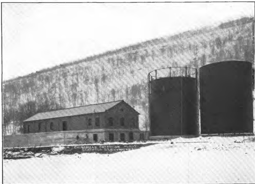
A. WATER AND AIR STORAGE TANKS.
