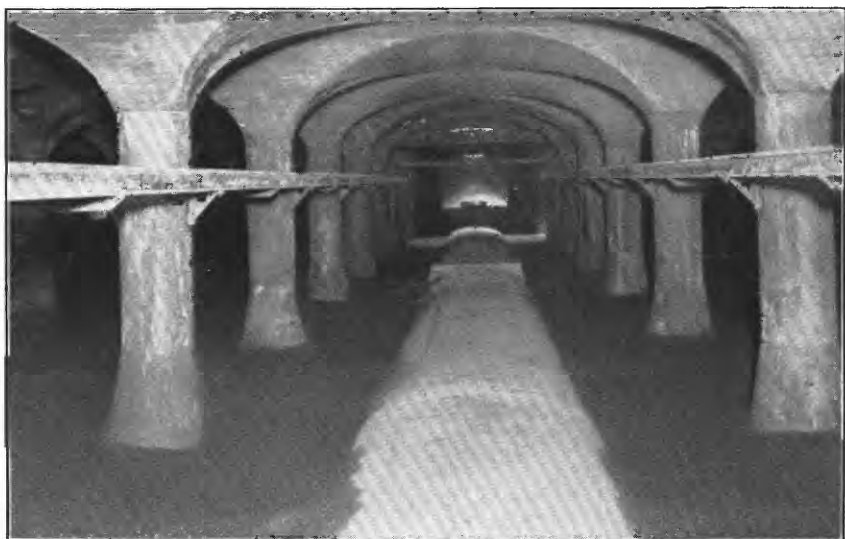
B. MAIN COLLECTOR AND LATERALS, WITH GRAVEL IN PLACE.
