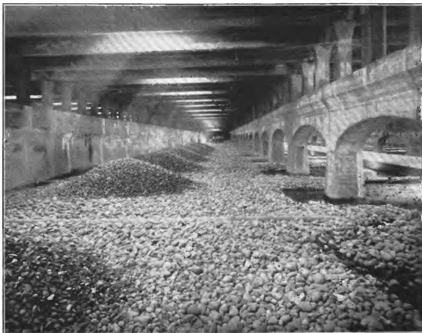
A. QUEEN LANE PLANT, WITH COARSE GRAVEL IN PLACE.
