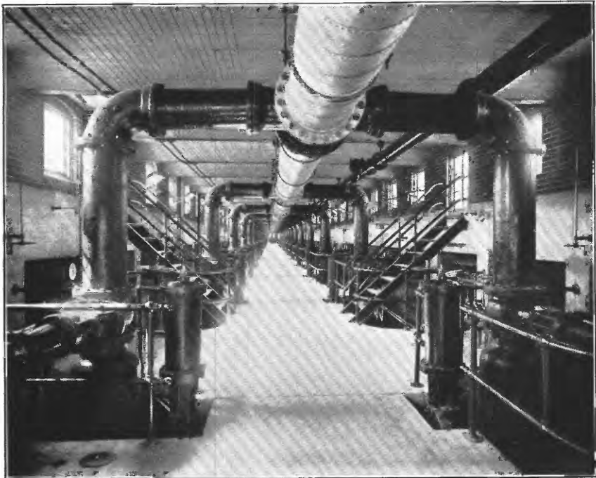
A. OPERATING GALLERY OF THE TORRESDALE PREFILTER, PHILADELPHIA, PA.
