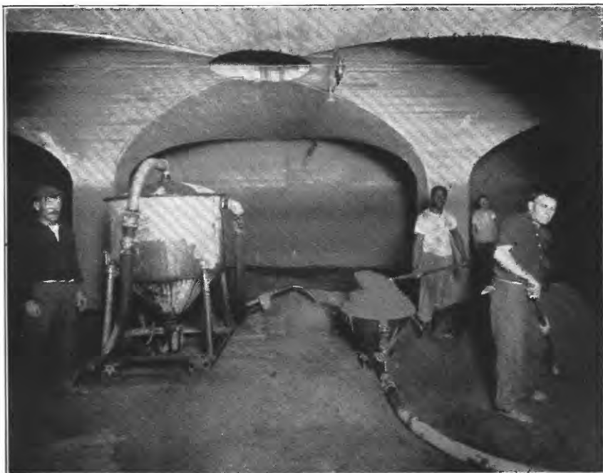
B. TORRESDALE PLANT, SHOWING METHOD OF CLEANING WITH NICHOLS SEPARATOR.
