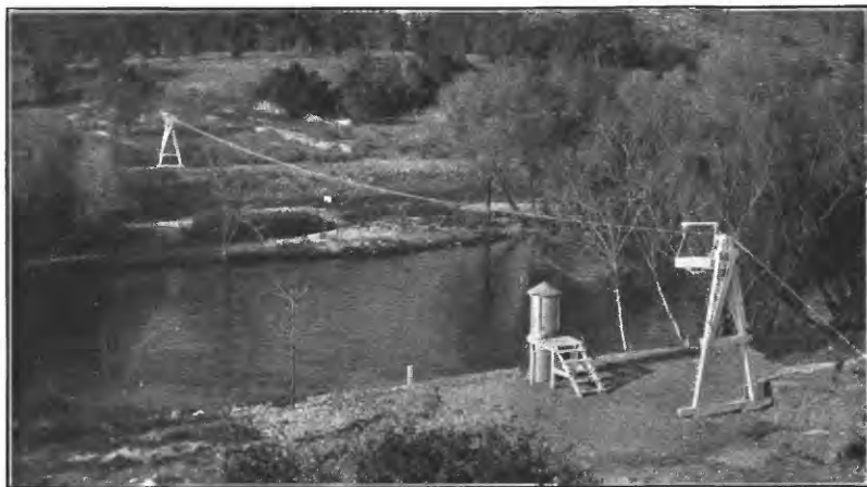
B. RECORDER HOUSE AND MEASURING CABLE ON KAWEAH RIVER, THREE RIVERS, CALIF.
