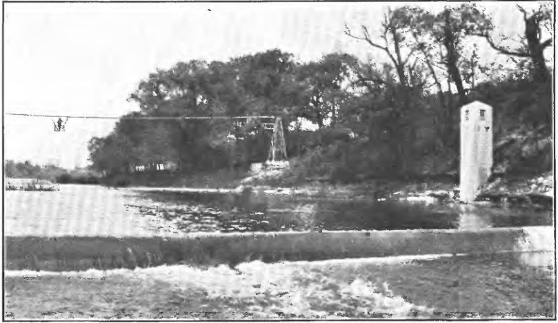
A. ARTIFICIAL CONTROL, RECORDER HOUSE, AND MEASURING CABLE ON OLEN-TANGY RIVER, DELAWARE, OHIO.
