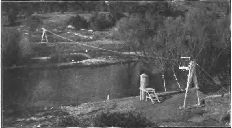
B. RECORDER HOUSE AND MEASURING CABLE ON KAWEAH RIVER, THREE RIVERS, CALIF.
