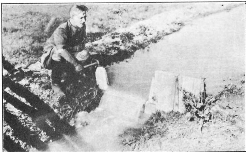
B. MEASURING THE DISCHARGE FROM WELL (D-5-1)8dc DURING A TEST OF INTERFERENCE WITH OTHER WELLS.
