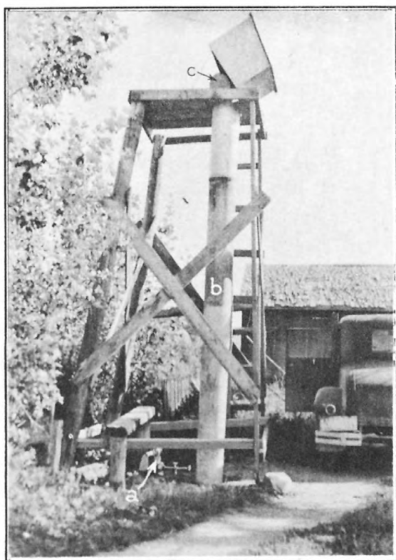
A. INSTALLATION OF AN AUTOMATIC WATER-STAGE RECORDING GAGE ON FLOWING WELL (D-5-1)17ac5.
