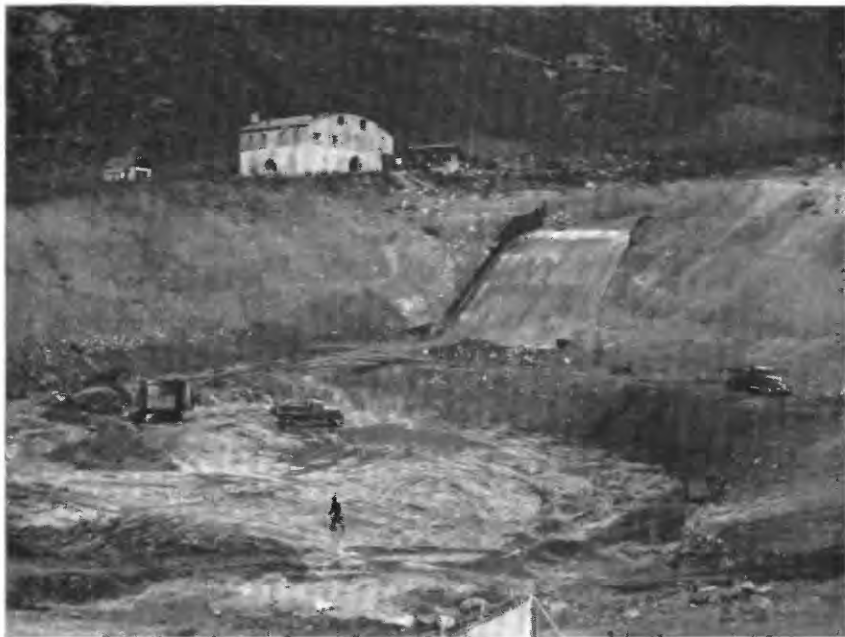
A. EXCAVATED BASIN AND INFLOW STRUCTURE.
