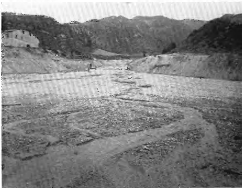
A. VIEW UPSTREAM SHOWING DEBRIS DEPOSITS UP TO ALTITUDE OF INFLOW STRUCTURES.
