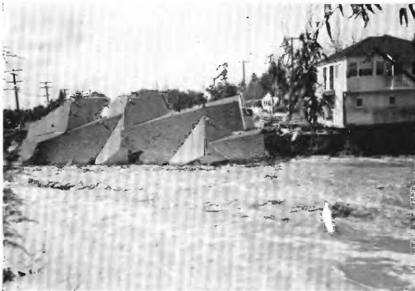
A. DESTRUCTION BY MEANDERING STREAM. Note composition of stream banks.
