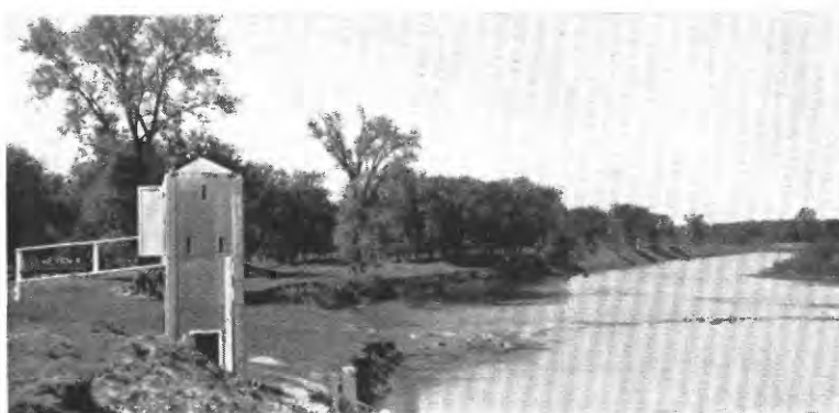
C. MINNESOTA RIVER NEAR CARVER, MINN. GAGING-STATION STRUCTURES.
