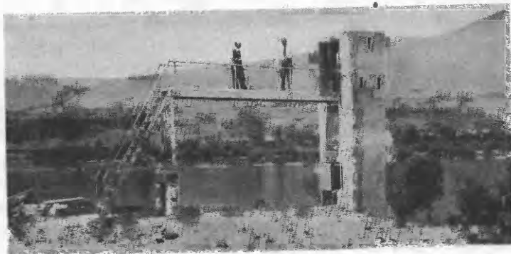
B. COLUMBIA RIVER NEAR THE DALLES, OREG. Gage shelter and stilling well.
