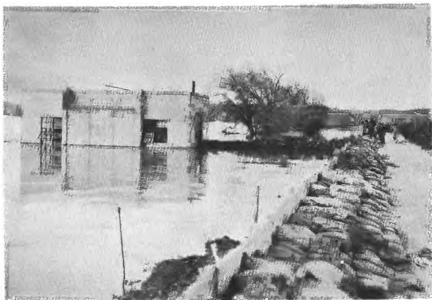
Figure 21.--Emergency levee built on existing levee at the intake structure of Council Bluffs. Photograph by Council Bluffs Nonpareil.
