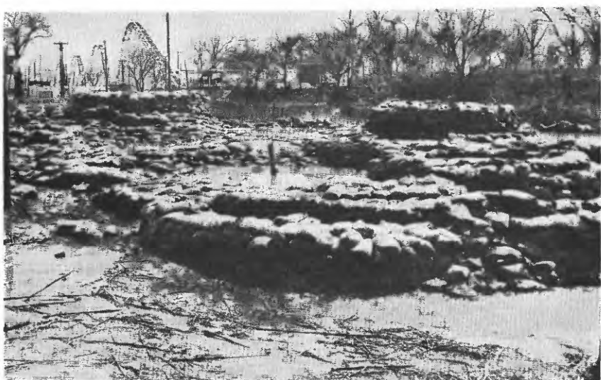
Figure 22. --Sand boils controlled by ring dikes of sandbags behind Council Bluffs levee. Photograph by Council Bluffs Nonpareil.
